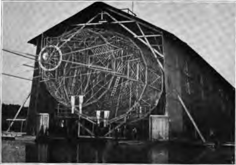
THE METAL SKELETON OF THE DIRIGIBLE "ZEPPELIN"
