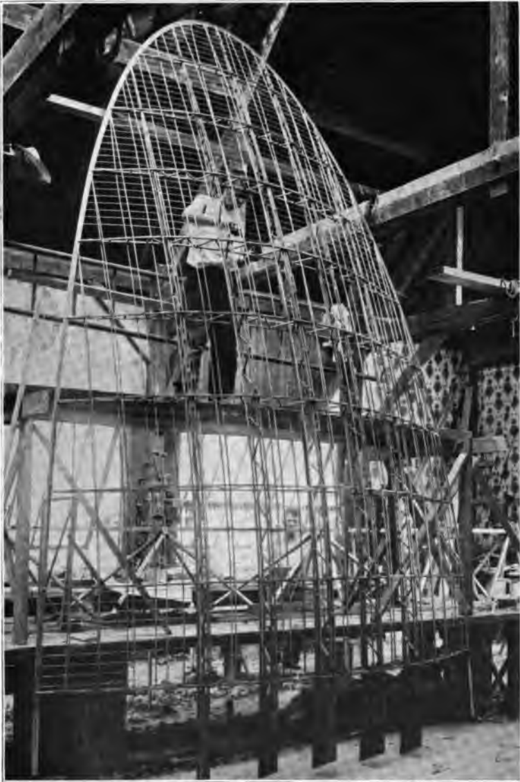
CONSTRUCTING AN AEROPLANE WING (FERBER)
